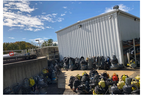
By streamlining their inventory, the Suffolk County DPW realizes a cost avoidance of $24,000 versus having multiple controllers on the shelf.
