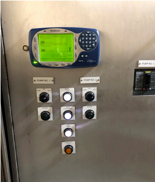
Along with the Flygt Outpost SCADA system, Suffolk County DPW installed Xylem's MultiSmart® Pump Station Managers (iPSM) to simplify its waste and sewage water management processes.
